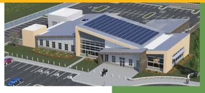
systems to determine which is the best performing and most cost effective for the expected life of the building. A large photovoltaic array will provide over 60,000 kWh of energy annually and contribute to Samaha meeting the "2030 Challenge" adopted by Loudoun County with achieving greater than 60% energy savings beyond established ASHRAE standards.
